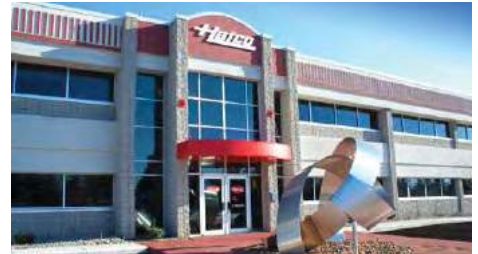
Sturgeon Bay - Manufacturing Facility 208 East Deck Street | Sturgeon Bay, WI 54235 920-743-5595
